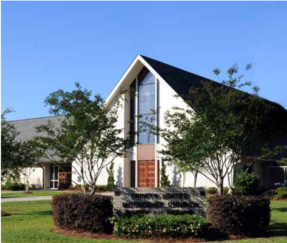
After Katrina, Trinity United Methodist Church in Gulfport, Mississippi had little physical damage, but 90% of the houses in the vicinity were flooded from one-to-eight feet. Photo by Tommy Triplett
